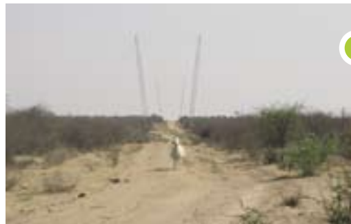
A ground transect that is cleared of bush and trees and provides easy access to the powerline, yet does not interfere with farming operations, is an essential requirement of NamPower.
